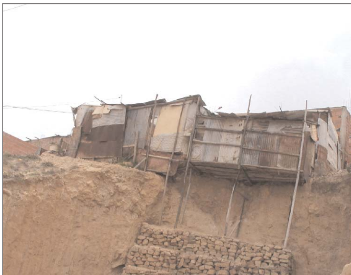
Some of the houses in Los Cerros del Sur are propped up by posts as the hillside below it erodes away. An earthquake in the area would be disastrous.
